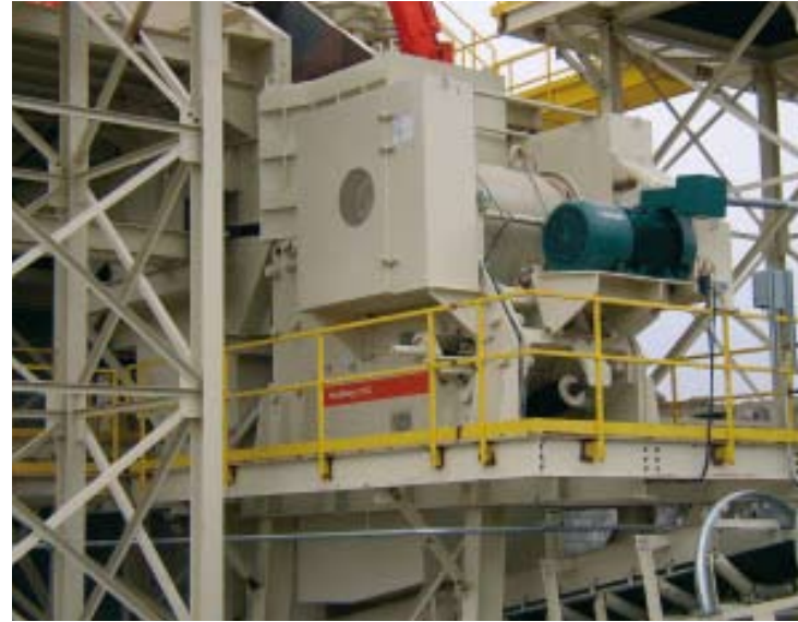
A C145 during the installation phase at a new primary crushing plant.
